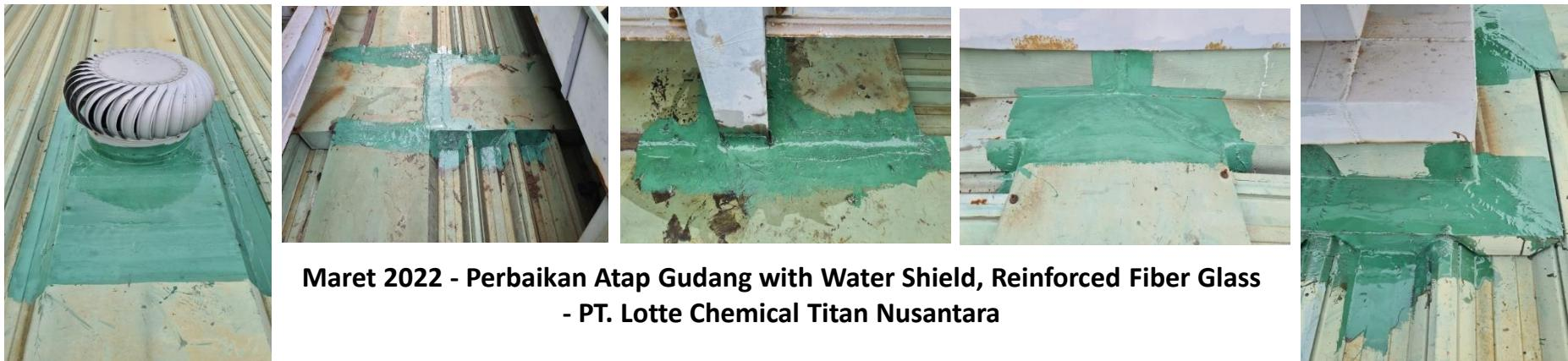
Maret 2022 - Perbaikan Atap Gudang with Water Shield, Reinforced Fiber Glass
